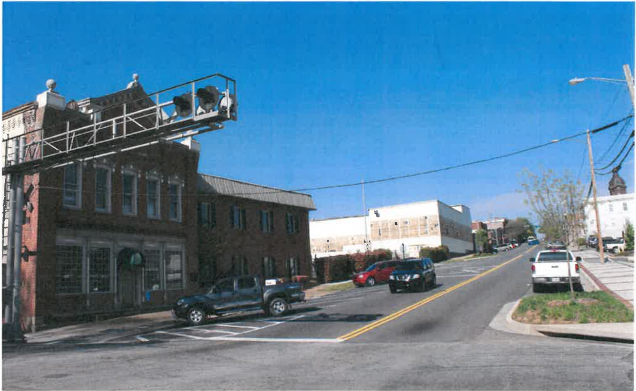
Figure 7i: Current condition at East Broad Street (looking west)
